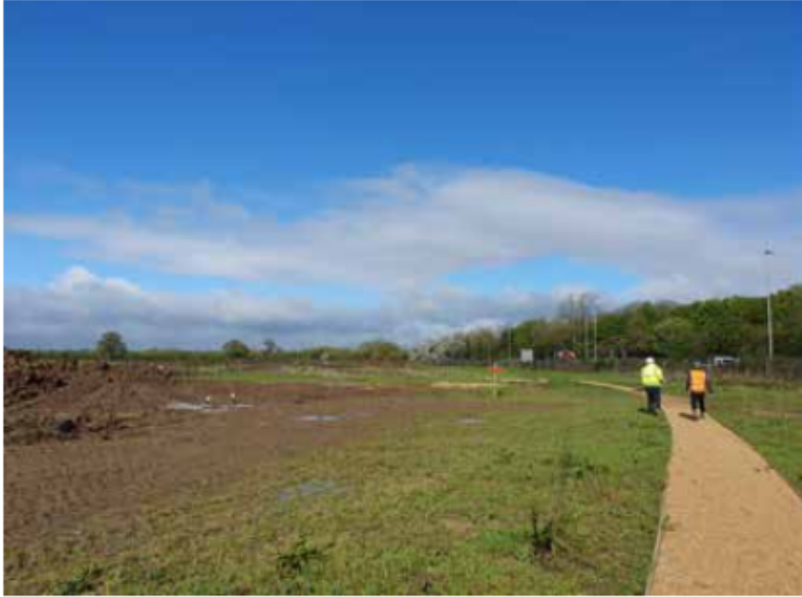
Site Photo A
